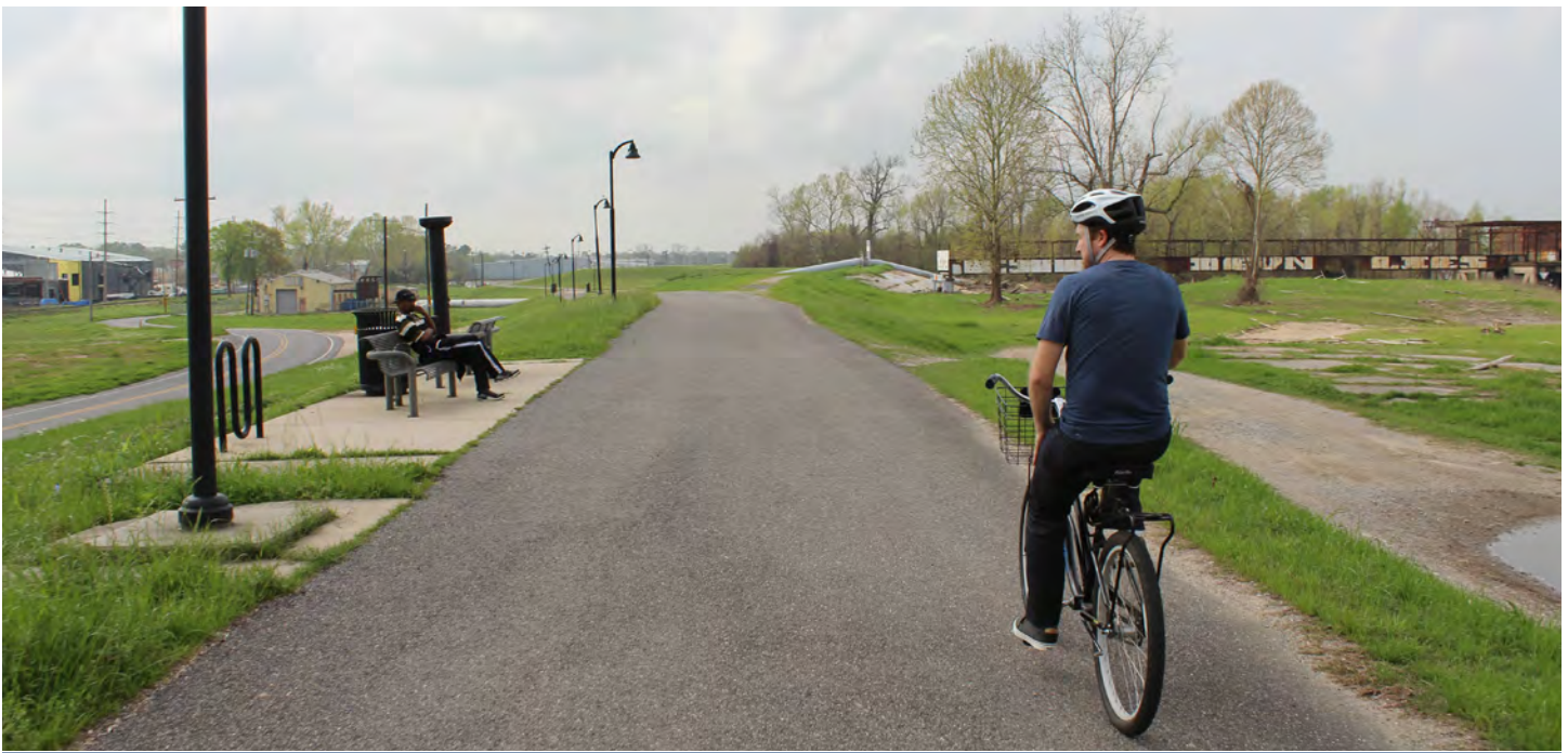
Figure 5: Mississippi River Levee Trail provides a continuous connection between Downtown and LSU
