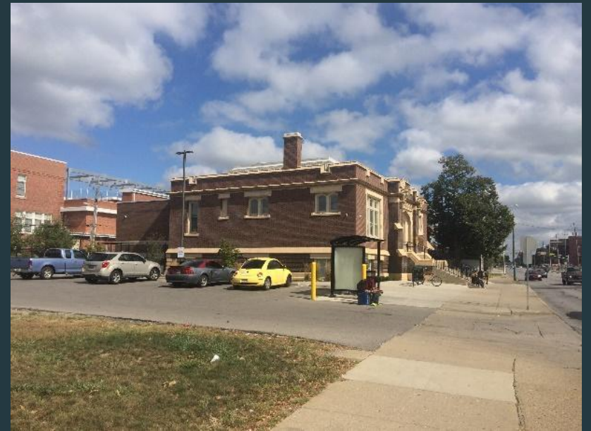
Washington and Rural; near future BL station
