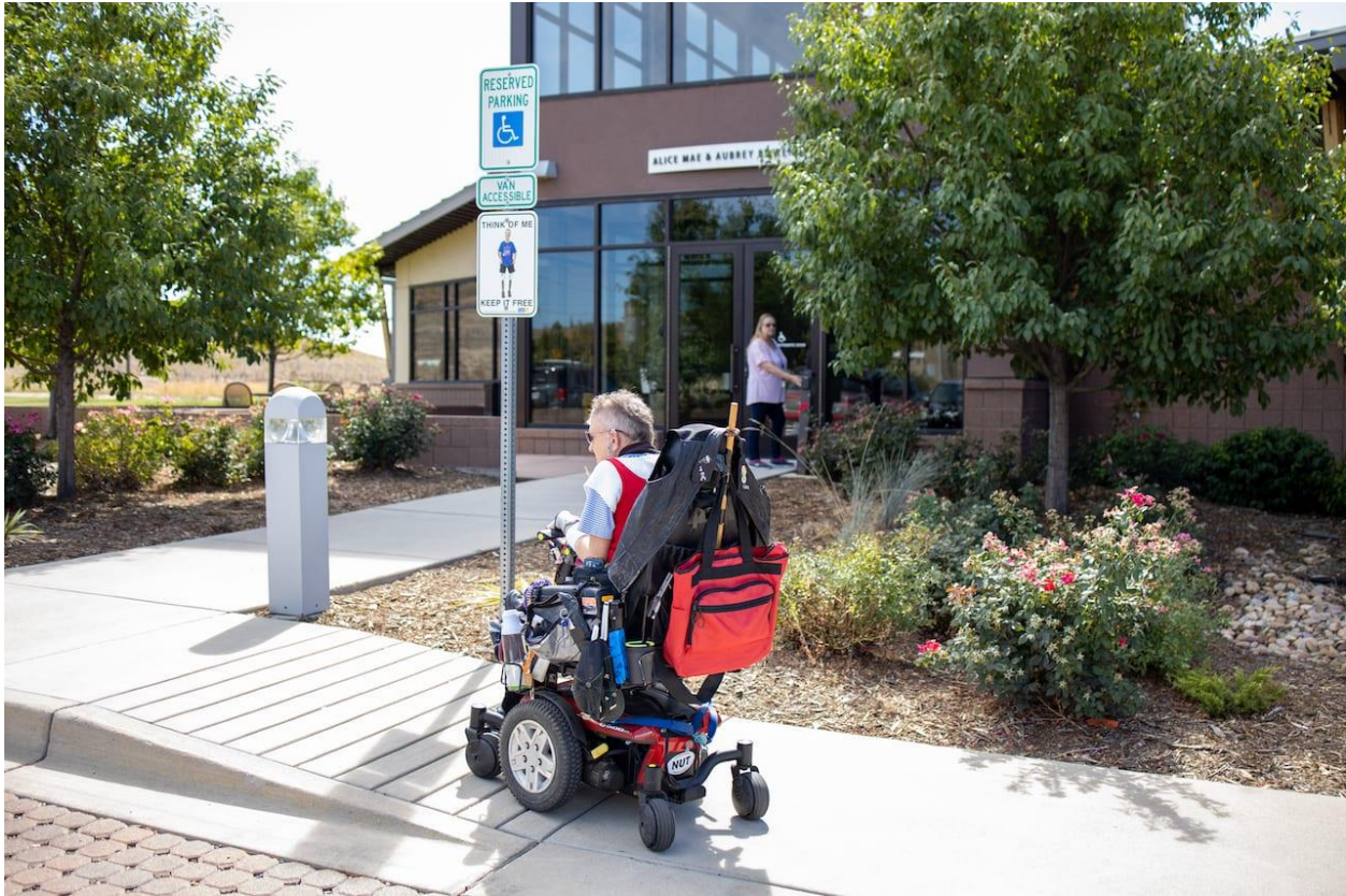
Figure 8: Woman in powerchair using curb cut that is marked with handicapped sign and truncated domes | Source: NADTC
