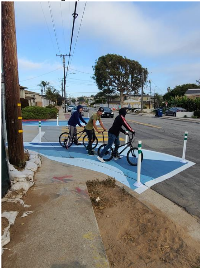
Figure 5: Three teenagers riding bikes on a curb bump-out installation which creates a barrier from vehicle traffic |Source: Street Plans
