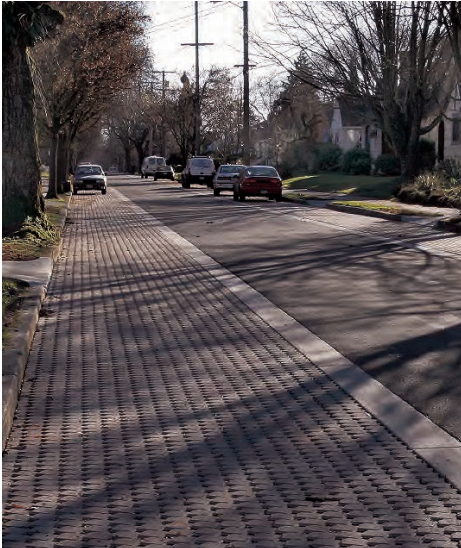
Pervious pavers for Water Quality
