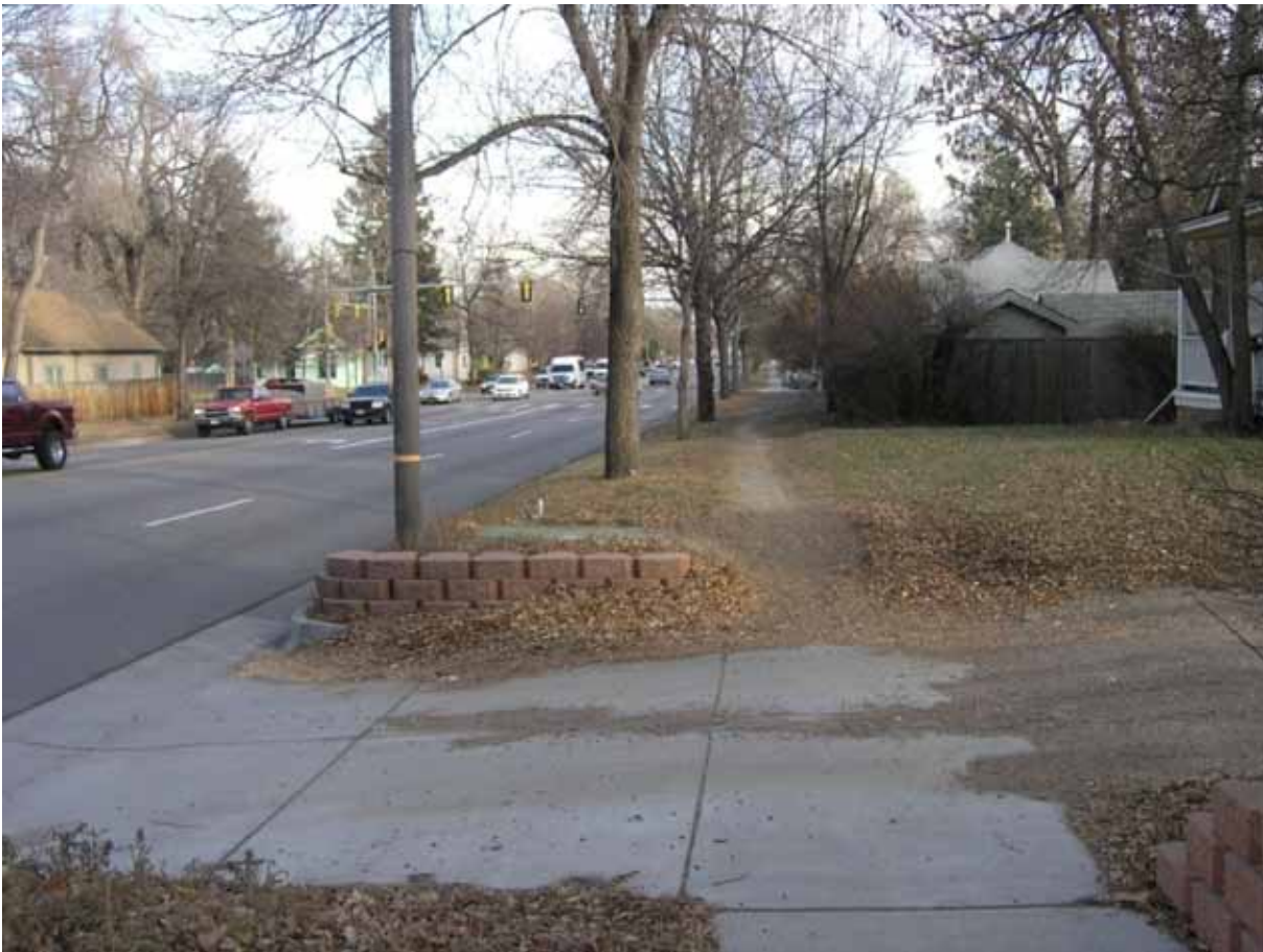
Example of existing gap in sidewalk system
