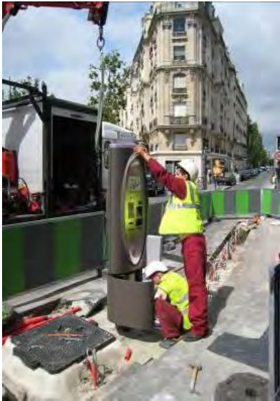
Figure 11 - Construction of a Vélib station in Paris
