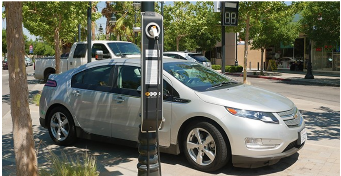
Streetlight Charging Station
