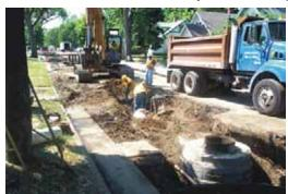
Minneapolis proactively began a sewer separation program to provide adequate system capacity and minimize overflows. Source: City of Minneapolis Public Works
