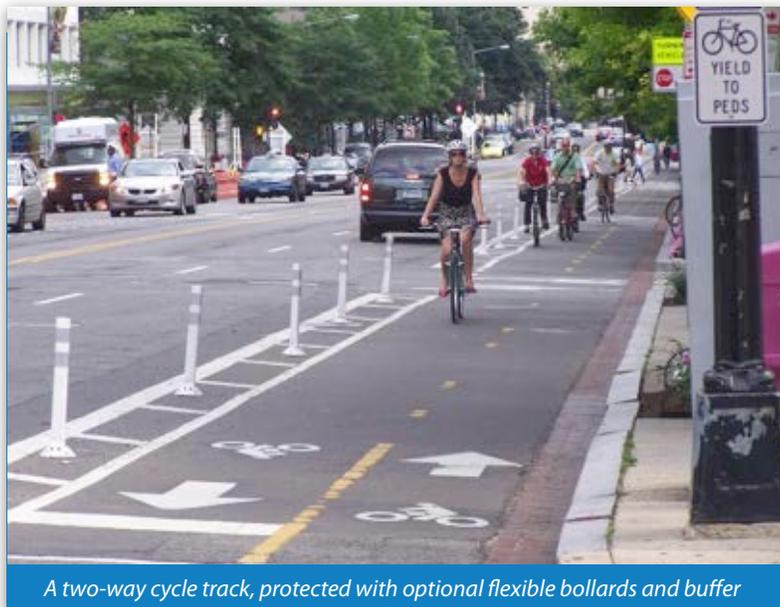
*A two-way cycle track, protected with optional flexible bollards and buffer*
