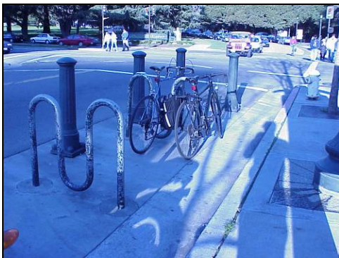
Clustered racks in a car parking space protected by bollards (Berkeley, CA).
